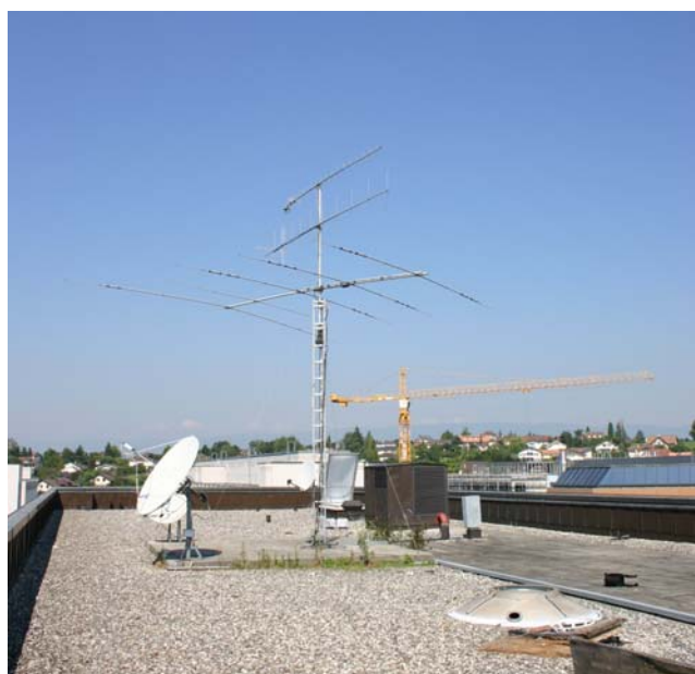
Figure V-4: Current installation on the roof of the EL building.
